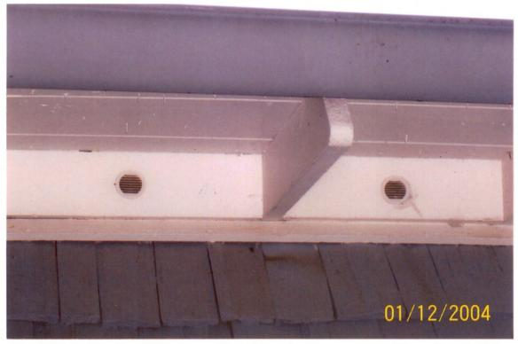
Fascia Vent. Fascia vents are usually only used with an open soffit, such as in this picture.
