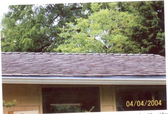
Ridge Vent # 1. Because the cathedralized roof was not vented properly with a ridge vent, moisture has damaged the plywood on this roof.
