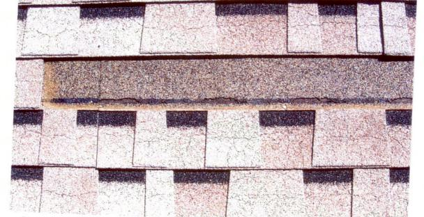
Sometimes heat-damaged shingles will have long cracks in the sningles surrace, called "Crazing"
