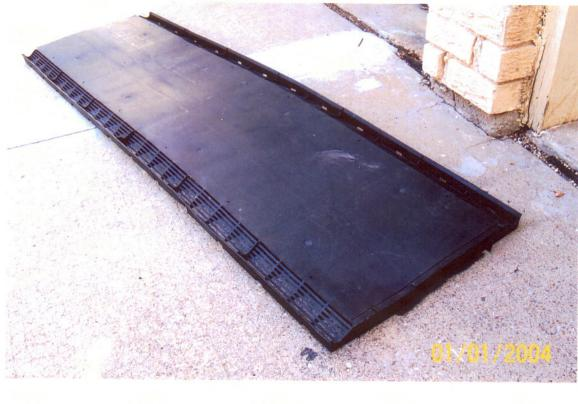
Baffled? A Baffled Ridge vent.
