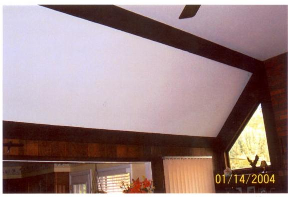
Cathedralized # 2. A partially cathedralized roof does not require ridge venting specifically. Gravity vents will do fine.
