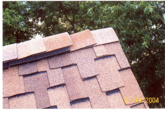
Ridge Vent # 3. Ridge vents should end about 1 foot away from the end gable (more with open soffits).
