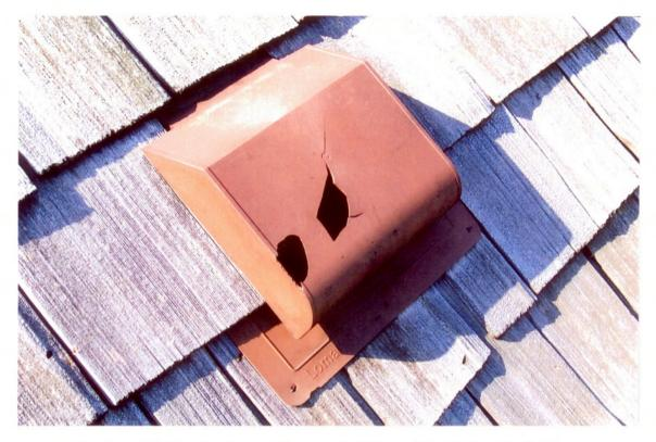
Shattered! This plastic vent became brittle and broke in a hailstorm.
