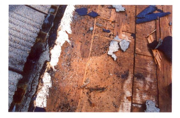
Wood Rot: Moisture build-up can severely damage plywood
