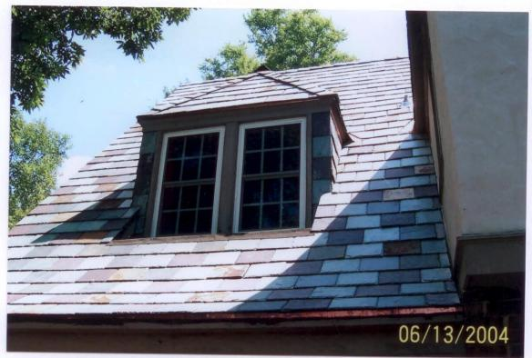
Picture #7 We can even use Tru-Slate on dormer sidewalls.
