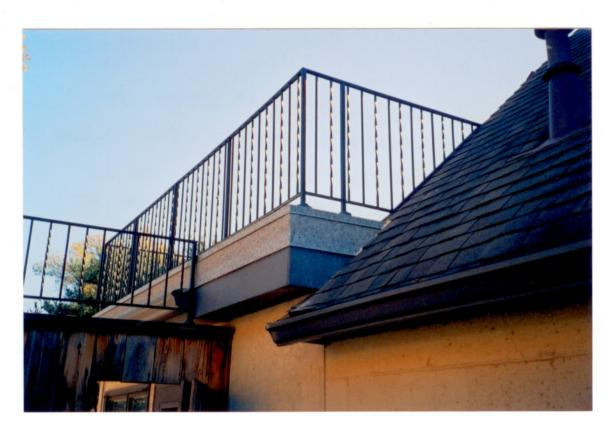
Picture #8 The roof level was raised to create proper drainage. We covered the unfinished edge with the same custom flatroofing and tied it into custom flashings.
