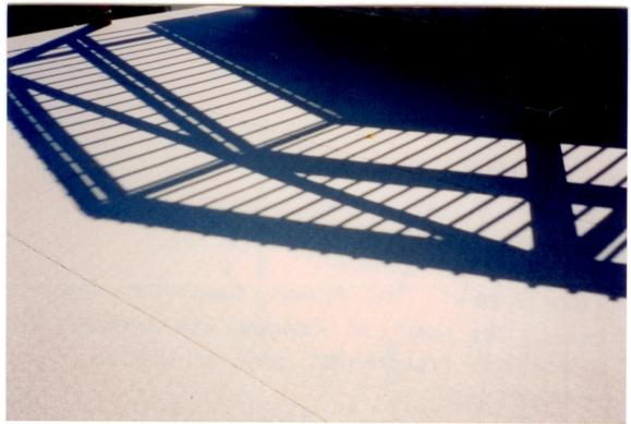
Picture #5 Dec-tec detail. In this picture, you can see the seams because the sun is casting hard shadows. This picture shows that even under the worst of lighting circumstances, a properly constructed seam is visually inconspicuous.
