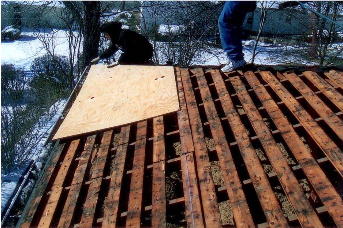
Photo #7 Because the eighth board has been moved, so the top edge of the plywood sheet has a slat beneath.
