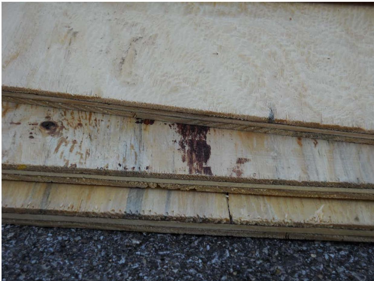
Photo #2 We can see the plied layers of CDX on the side profile.
