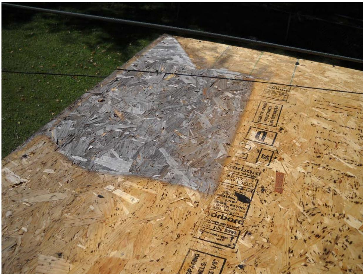
Photo #5 OSB really does hold up to water exposure nowadays.
