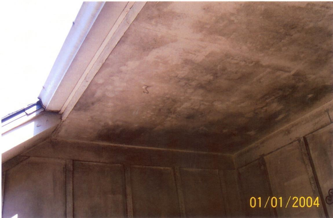
**Mold: A moldy soffit. This kind of mold is usually due to ventilation problems.**
