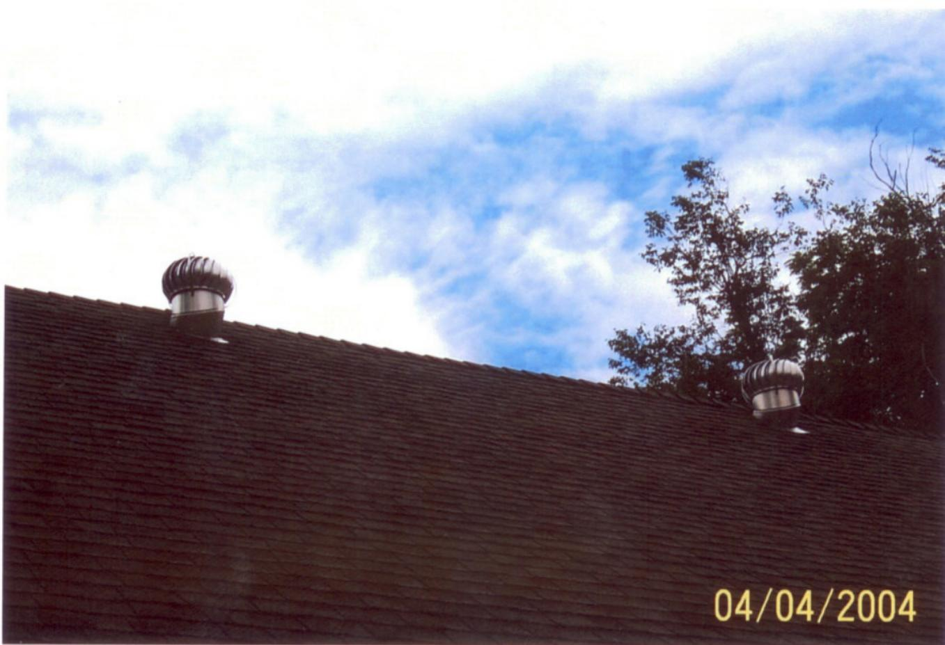
**Turbines. Spinning turbines used to be the preferred ventilation product.**
