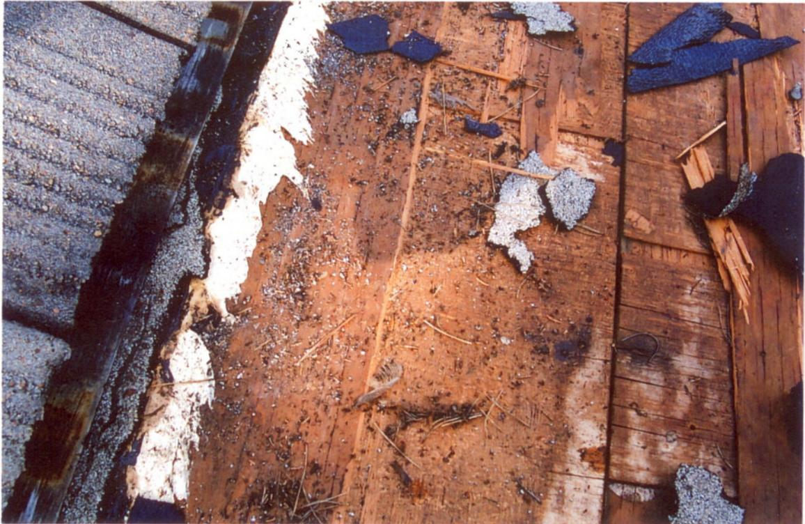
**Wood Rot: Moisture build-up can severely damage plywood**
