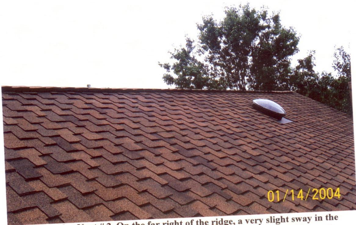
**Ridge Vent # 2. On the far right of the ridge, a very slight sway in the roofline has transposed into a noticeable downward twist in the ridge vent.**
