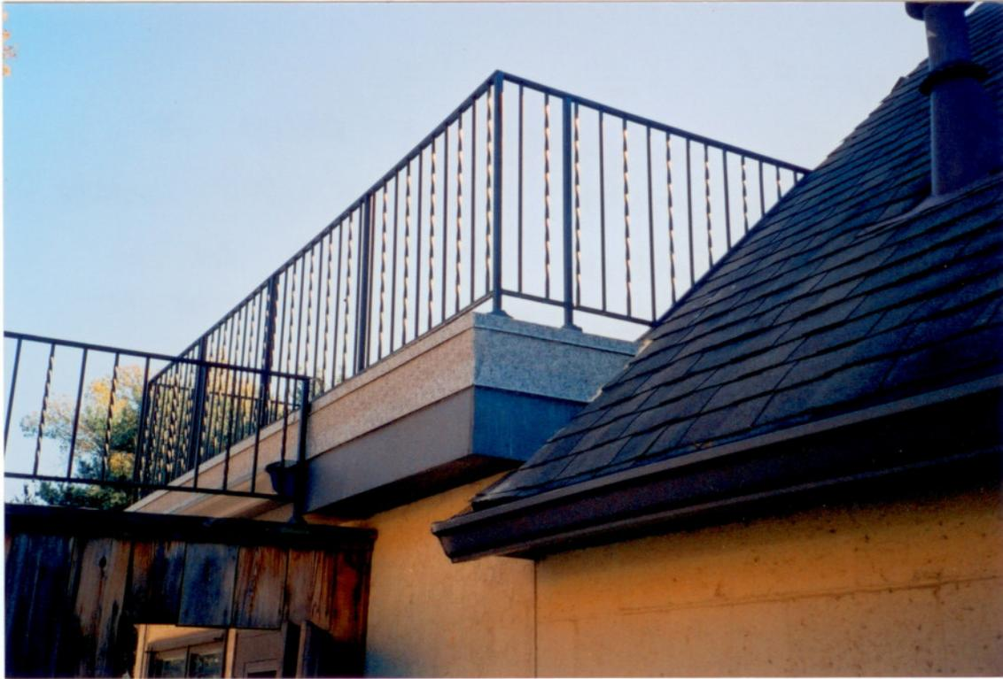
**Picture #8 The roof level was raised to create proper drainage. We covered the unfinished edge with the same custom flatroofing and tied it into custom flashings.**
